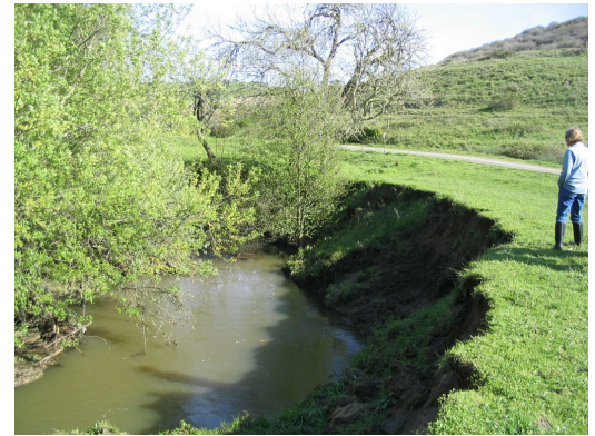
Creek bank erosion before restoration planting
